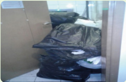
Blocked access and fire risk
